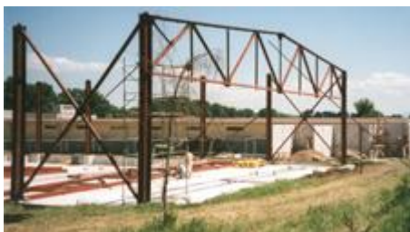
Picture: Construction of a pharmaceutical production plant in Bulgaria (2006, PSOM)
